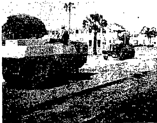
The roads are getting their long-overdue "face lift," as shown by the resurfacing of Clinton and Borden.
