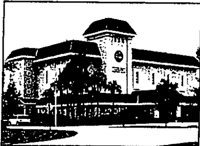
The Southern Region Water Reclamation Facility is an integral component in the County's water conservation program. It is a state-of-the-art wastewater treatment facility that produces reclaimed water used for irrigating lawns and golf courses.
