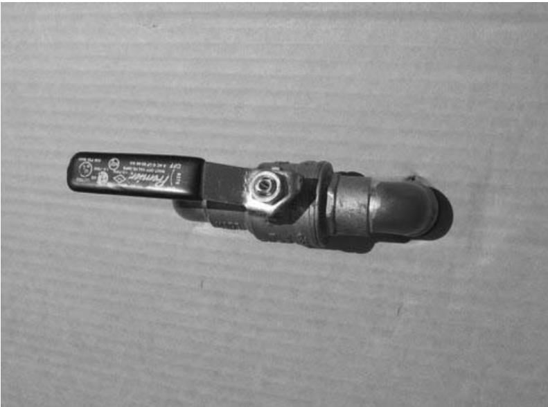
Top view of shutoff valve. See side view on Page 1. Photo by Dan Gladstone
