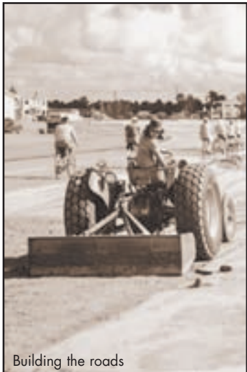
Building the roads
