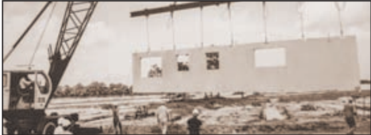
First in Florida – using pre-fabricated building materials
