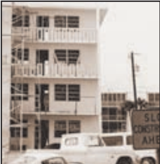
4-story building construction underway
