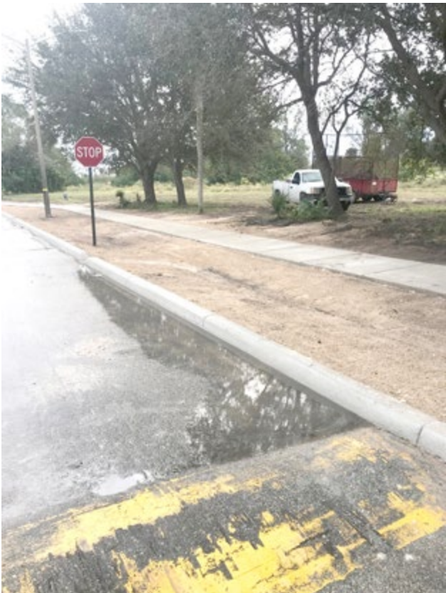
AT THIS SPOT, RAINWATER IS COLLECTING AT JUNCTURE OF NEW CURB AND OLD SPEED BUMP. THIS IS A “PUNCH LIST” ITEM THAT WILL BE CORRECTED WITH AN ADDITIONAL CURB CUT. CROSSWALKS, STRIPING, AND SPEED BUMPS WILL BE REPAINTED IN JANUARY.
