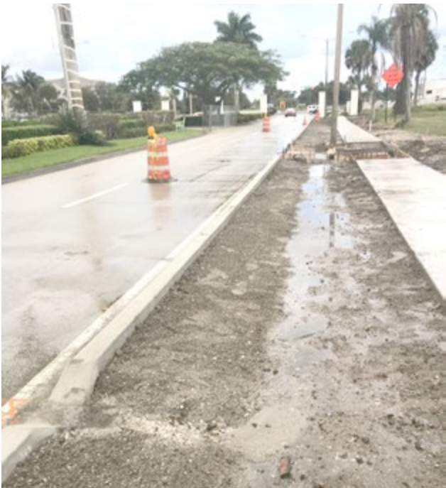
CURB AND SIDEWALK INSTALLATION COMPLETE. AFTER THE FIRST BIG RAINSTORM, WATER IS DRAINING NICELY FROM ROADWAY TO DRAINAGE SWALE.
