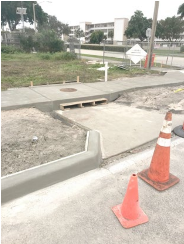
INSTALLATION OF DRAINAGE FLUME COMPLETE. THERE ARE TWO OF THESE, AT THE EAST AND WEST ENDS OF THE NEW WALKWAY.
