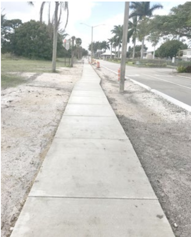
NEW SIDEWALK OPENED ON 12/25. NEXT JOBS ARE INSTALLATION OF FENCE, IRRIGATION, AND SOD. SIDEWALK IS CLOSER TO PROPERTY LINE THAN TO ROADWAY-THIS IS FOR PEDESTRIAN SAFETY, AND TO ALLOW RAINWATER TO DRAIN FROM ROADWAY TO DRAINAGE SWALE BETWEEN SIDEWALK AND CURB.
