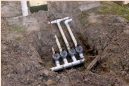
IRRIGATION CONTROL VALVES AT CV RESIDENTIAL BUILDING- THIS IS WHERE UCO RESPONSIBILITY ENDS AND ASSOCIATION'S BEGINS.
