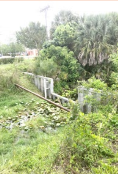
THIS STATIONARY WEIR (A TYPE OF DAM), IS LOCATED AT SOUTH SIDE OF CENTURY VILLAGE AND HOLDS IN THE PROPERTY’S STORED IRRIGATION WATER. WHEN WATER LEVEL REACHES TOP OF DAM, EXCESS WATER MOVES OVER DAM INTO DRAINAGE CANAL OWNED BY LAKE WORTH DRAINAGE DISTRICT. THIS USUALLY ONLY HAPPENS DURING STORMS.
