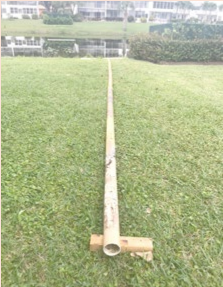
IRRIGATION WATER INTAKE PIPE- THESE NEED TO BE PERIODICALLY PULLED FROM LAKE AND CLEANED.
