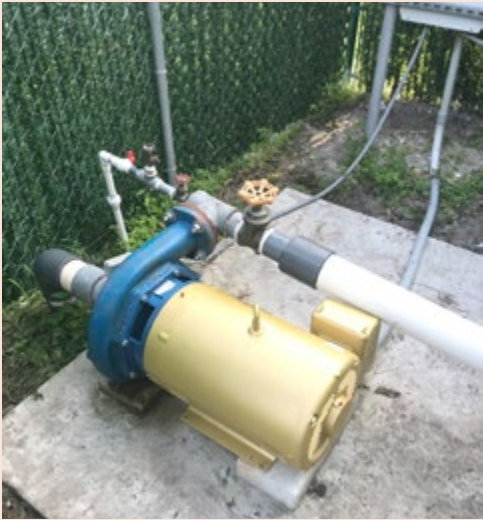
THIS IRRIGATION PUMP STATION, ONE OF TWENTY-TWO, PULLS IRRIGATION WATER FROM CV WATERWAYS.
