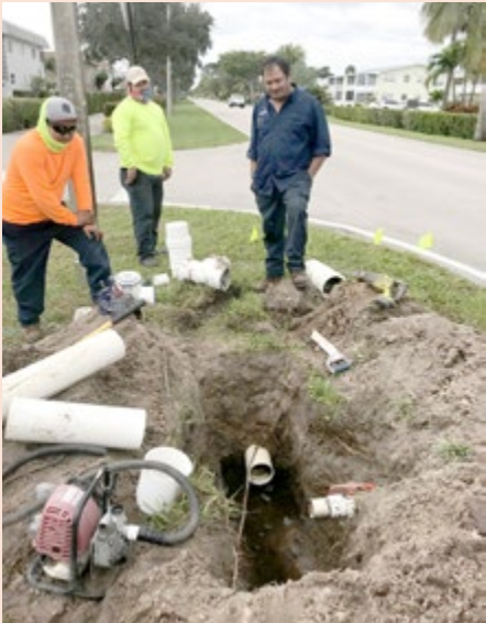
IRRIGATION MAINLINE PIPES ARE JUST UNDER SURFACE OF GRASS- THIS DAMAGE, ALONG NORTH DRIVE, WAS LIKELY CAUSED BY VEHICLES PULLING OFF ROAD ONTO GRASS.
