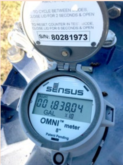
INCOMING RECLAIMED WATER IS METERED BY PALM BEACH COUNTY WATER UTILITIES. BILL IS SENT TO UCO.
