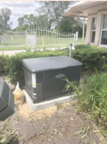
HAVERHILL ROAD ENTRANCE- NEW EMERGENCY GENERATOR WILL PROVIDE UNINTERRUPTED POWER TO GUARDHOUSE, GATE ARM, AND LIGHTS.
