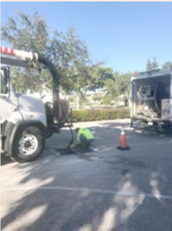
KENT SECTION- CONTRACTOR CLEANING AND INSPECTING STORM DRAIN PIPE. APPROXIMATELY ONE HALF OF ALL CV STORM DRAIN PIPES WERE CLEANED/INSPECTED IN 2019.
