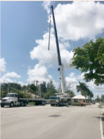
WEST DRIVE- NEW CONCRETE UTILITY POLE BEING LOWERED INTO PLACE.
