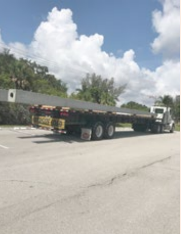
WELLINGTON SECTION- NEW CONCRETE UTILITY POLE READY FOR INSTALLATION
