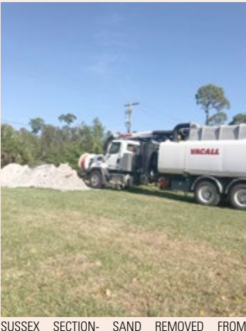
SUSSEX SECTION- SAND REMOVED FROM STORM DRAIN PIPES, PILED UP FOR REMOVAL OFF PROPERTY. CLEAN STORM DRAIN PIPES MEAN FASTER DRAINAGE OF ROADS DURING MAJOR STORMS.
