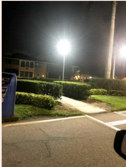
CENTURY BOULEVARD- LED FIXTURE INSTALLED TO LIGHT UP PEDESTRIAN CROSSWALK AT MEDIAN.
