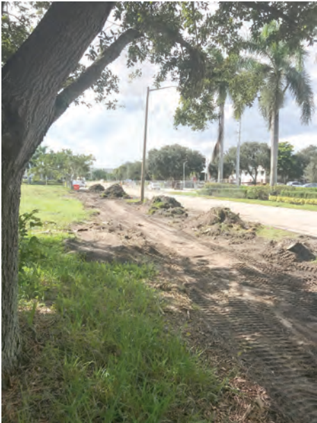
10/24- OLD SIDEWALK AND SOD REMOVED, ROUGH GRADING BEGUN.
