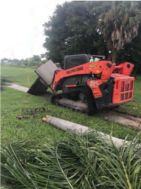
10/23- OLD SIDEWALK BEING REMOVED.
