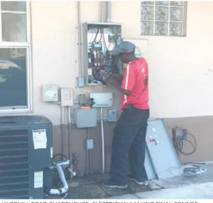
HAVERHILL ROAD GUARDHOUSE- ELECTRICIAN MAKING FINAL CONNECTIONS FOR NEW EMERGENCY GENERATOR.
