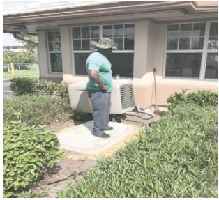
OKEECHOBEE BOULEVARD GUARDHOUSE- 2/27, NEW EMERGENCY GENERATOR BEING INSTALLED ON A PRECAST CONCRETE BASE.
