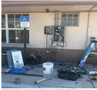
OKEECHOBEE BOULEVARD GUARDHOUSE- ELECTRIC SERVICE PANEL AND TRANSFER SWITCHGEAR FOR NEW GENERATOR INSTALLED.
