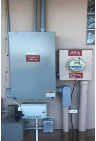
HAVERHILL ROAD GUARDHOUSE- AUTOMATIC TRANSFER SWITCH FOR EMERGENCY GENERATOR, MOUNTED ON THE WEST SIDE OF THE GUARDHOUSE. WHEN POWER GOES OUT, THERE IS A SHORT DELAY, THEN THIS SWITCH AUTOMATICALLY LOCKS OUT MAINS POWER (FPL) AND STARTS THE EMERGENCY GENERATOR. WHEN MAINS POWER RETURNS, THE SEQUENCE IS REVERSED. THIS IS AN IMPORTANT SAFETY FEATURE.
