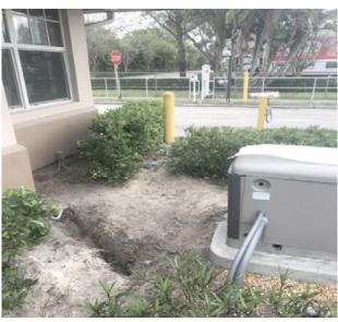
OKEECHOBEE BOULEVARD GUARDHOUSE- POWER CABLES BETWEEN NEW GENERATOR AND BUILDING ARE INSTALLED.
