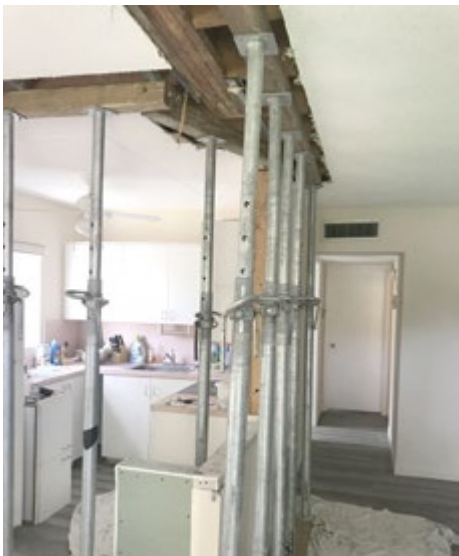
NORWICH SECTION- FLOOR JACKED UP, NINE BRACES IN PLACE.
