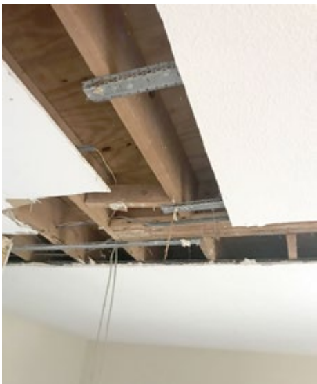
NORWICH SECTION- CONTRACTOR REMOVES CEILING OF LOWER UNIT TO MAKE INSPECTION. FLOOR JOISTS ARE BOWED, DUE TO LACK OF SUPPORT BELOW.
