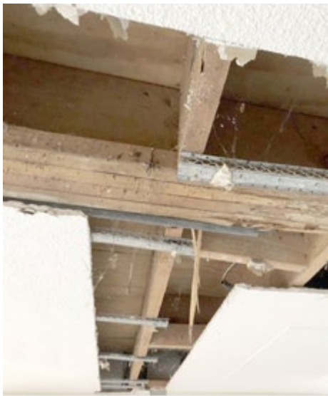
NORWICH SECTION- THE TERMITE DAMAGED FLOOR JOISTS MADE THE JACKING AND BRACING JOB MORE DIFFICULT- THE CONTRACTOR NEEDED TO FIND NON-DETERIORATED WOOD TO BRACE AGAINST.
