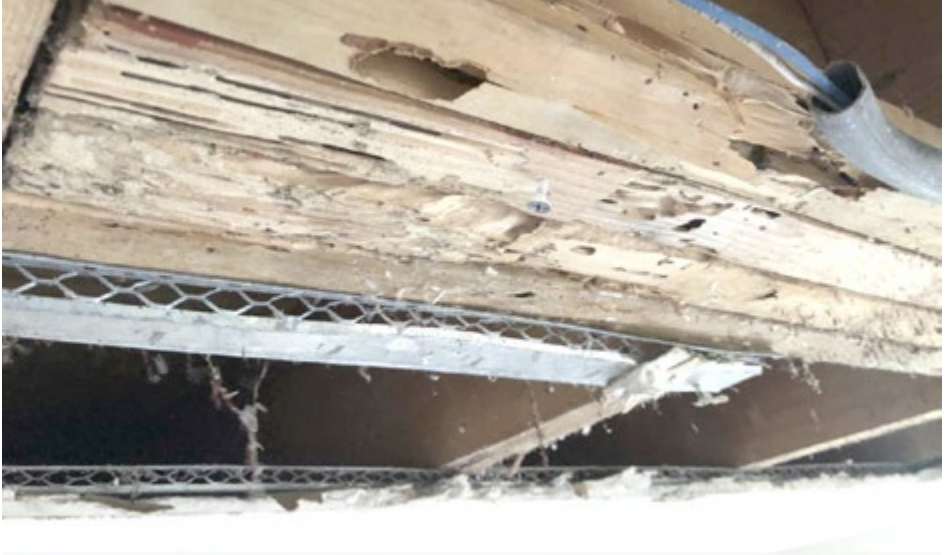
NORWICH SECTION- EXTENSIVE TERMITE DAMAGE AT FLOOR JOISTS. PREVIOUS REPAIR IS ALSO TERMITE DAMAGED. I WAS ABLE TO POKE HOLES THROUGH THE JOISTS WITH MY FINGER.
