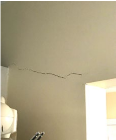
NORWICH SECTION- WALL CRACK AT UPPER UNIT EXTENDS INTO THE KITCHEN.
