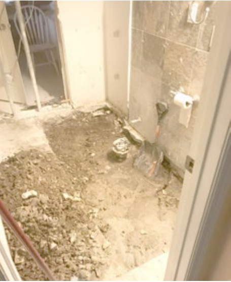
STRATFORD SECTION- CONCRETE SLAB FLOOR IS JACK HAMMERED UP AND REMOVED. THIS FLOOR IS CONDOMINIUM COMMON ELEMENT. THIS UNIT OWNER HAD NO BUSINESS DESTROYING PROPERTY THAT DOES NOT BELONG TO HIM.
