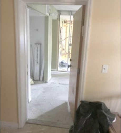
STRATFORD SECTION- UNPERMITTED, NON FIRE RATED DOOR INSTALLED BETWEEN THE TWO UNITS. THIS IS AN OBVIOUS FIRE HAZARD, AND, AGAIN, DESTRUCTION OF CONDOMINIUM COMMON PROPERTY.
