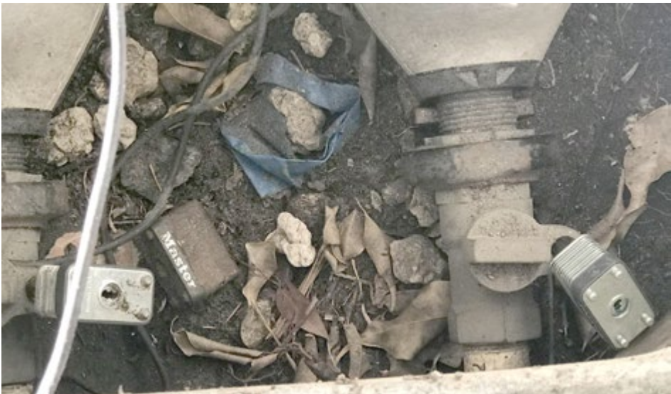
NORWICH SECTION- WATER SERVICES SHUT OFF AND LOCKED OFF BY PBC WATER UTILITIES TO DETER RE-OCCUPANCY BY UNIT OWNERS.
