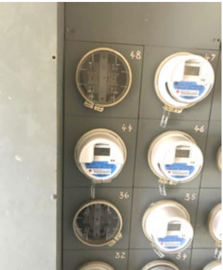
NORWICH SECTION- METERS AT BOTH UNITS PULLED BY FPL TO DETER RE-OCCUPANCY BY UNIT OWNERS.
