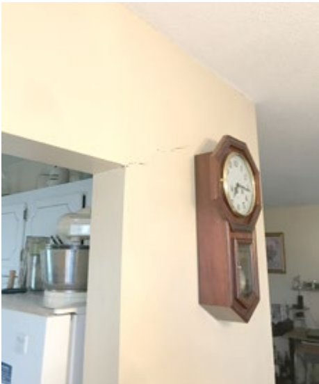
NORWICH SECTION- LARGE CRACK IN WALL. THE UPPER UNIT IS SUBSIDING.
