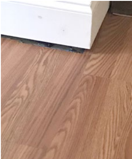
NORWICH SECTION- FLOOR AT UPPER UNIT SUBSIDED TWO INCHES, AND FLOOR FELT UNSTABLE UNDERFOOT. NOT GOOD.
