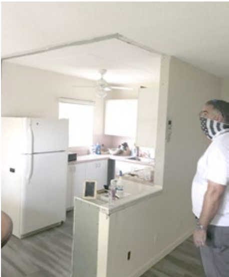
NORWICH SECTION- OWNER OF LOWER UNIT REMOVED LOAD BEARING WALLS FROM KITCHEN. NO PERMIT, NO PERMISSION FROM BOARD, SHODDY WORK PERFORMED BY AN UNLICENSED CONTRACTOR. UNIT OWNER WAS IN ECUADOR.
