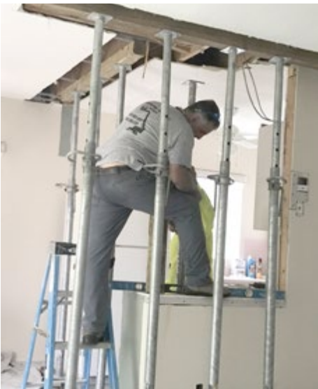
NORWICH SECTION- CONTRACTOR INSTALLS JACKS AND BRACES, BEGINS RAISING CEILING. THE TERMITE DAMAGED WOOD MADE THIS JOB MORE DIFFICULT.
