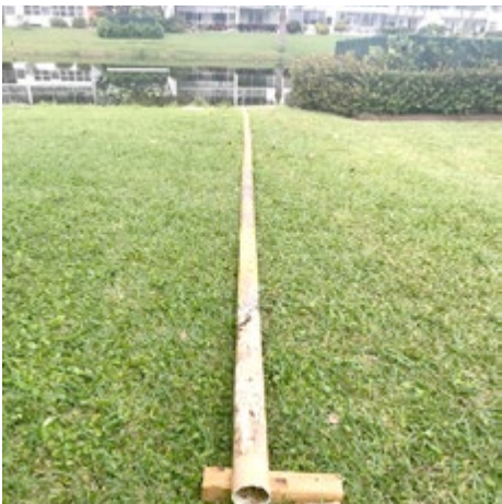
IRRIGATION WATER INTAKE PIPE- THESE NEED TO BE PERIODICALLY PULLED FROM LAKE AND CLEANED.
