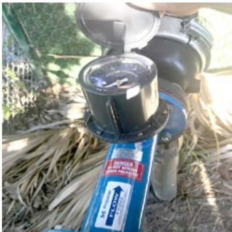
WATER PULLED FROM LAKE IS METERED- REPORT IS SENT TO SOUTH FLORIDA WATER MANAGEMENT DISTRICT EACH MONTH.
