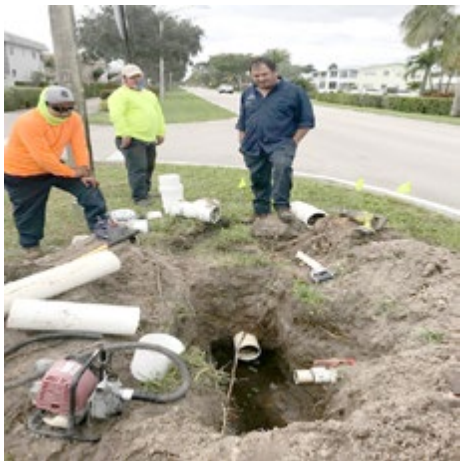
IRRIGATION MAINLINE PIPES ARE JUST UNDER SURFACE OF THE GRASS- THIS DAMAGE, ALONG NORTH DRIVE, WAS LIKELY CAUSED BY VEHICLES PULLING OFF ROAD ONTO GRASS.
