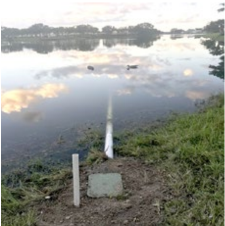
NORTH DRIVE- NEW SUCTION LINE AND CHECK VALVE INSTALLED BY CHABOT IRRIGATION ON 11/27/20. THE GREEN BOX CONTAINS A CHECK VALVE, WHICH KEEPS WATER MOVING IN ONE DIRECTION.
