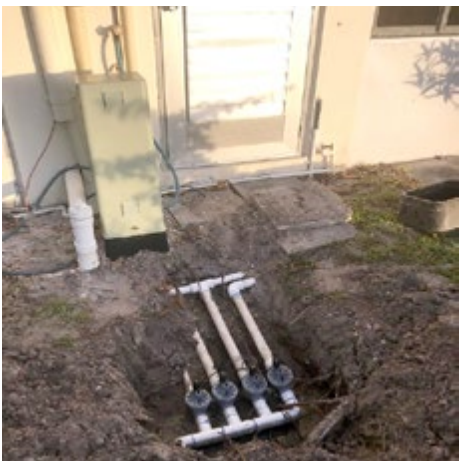
IRRIGATION CONTROL VALVES AT CV RESIDENTIAL BUILDING- THIS IS WHERE UCO RESPONSIBILITY ENDS AND ASSOCIATION'S BEGINS.
