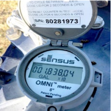
INCOMING RECLAIMED WATER IS METERED BY PALM BEACH COUNTY WATER UTILITIES. BILL IS SENT TO UCO.
