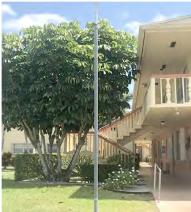
TREES THAT TOUCH THE BUILDING NEED TO BE TRIMMED BACK TO KEEP ROOF RATS OUT OF THE ATTIC, AND TO REDUCE THE RISK OF DAMAGE TO THE BUILDING DURING STORMS.
