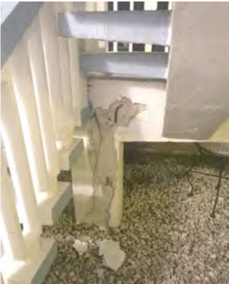
THIS STAIRCASE HAS BECOME UNSAFE. WATER HAS INTRUDED INTO THE CONCRETE, CAUSING REBAR SPALLING.
