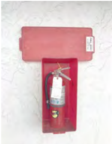
BUSTED FIRE EXTINGUISHER BOXES SHOULD BE NOTED AND RESOLVED BY THE MONTHLY PROPERTY MANAGER'S INSPECTION, BUT ANY UNIT OWNER CAN CALL THIS IN FOR REPAIR. THE NUMBER FOR THE FIRE EXTINGUISHER COMPANY IS ON THE TAG.
