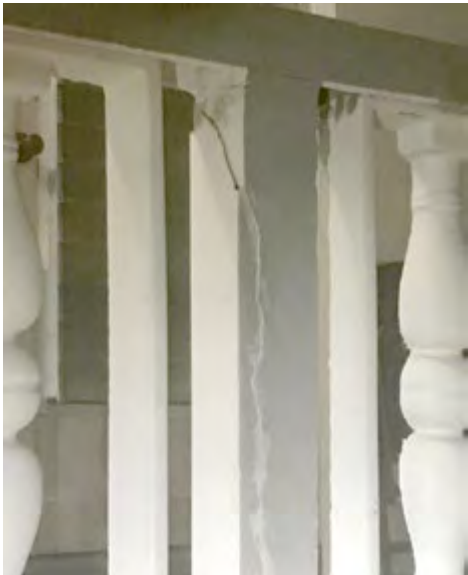
CRACKED BALUSTRADES ARE A COUNTY CODE VIOLATION, AND WILL BE NOTED ON THIS ASSOCIATION'S "REPORT CARD".
