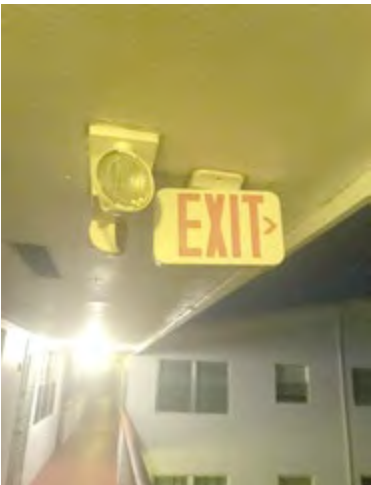
THIS IS A VERY COMMON "HIT" ON THE REPORT CARDS, NON FUNCTIONAL EMERGENCY LIGHTING. THIS IS MY OWN BUILDING. NOBODY'S REPORT CARD IS PERFECT.
