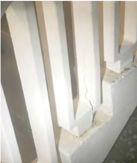
CRACKED RAILINGS AND BALUSTRADES NEED TO BE REPAIRED AS THEY ARE DISCOVERED. THE ASSOCIATION'S PROPERTY MANAGER SHOULD BE INSPECTING THIS BUILDING MONTHLY, AND PROVIDING A REPORT TO THE ASSOCIATION.
