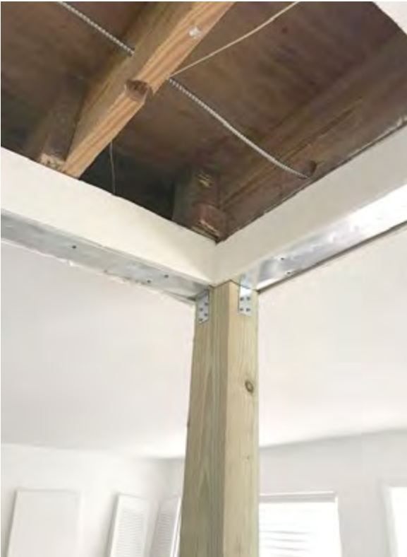
COVENTRY SECTION- THIS WOOD POST IS INTENDED TO BEAR THE LOAD PREVIOUSLY BORNE BY THE REMOVED INTERIOR WALL.
