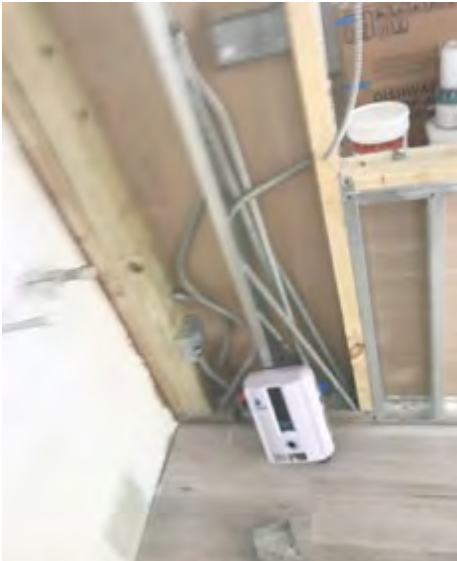
COVENTRY SECTION- TANKLESS WATER HEATER. THIS WAS NOT APPROVED BY THE BOARD AND COULD DANGEROUSLY OVERLOAD THE BUILDING'S ELECTRICAL WIRING.
