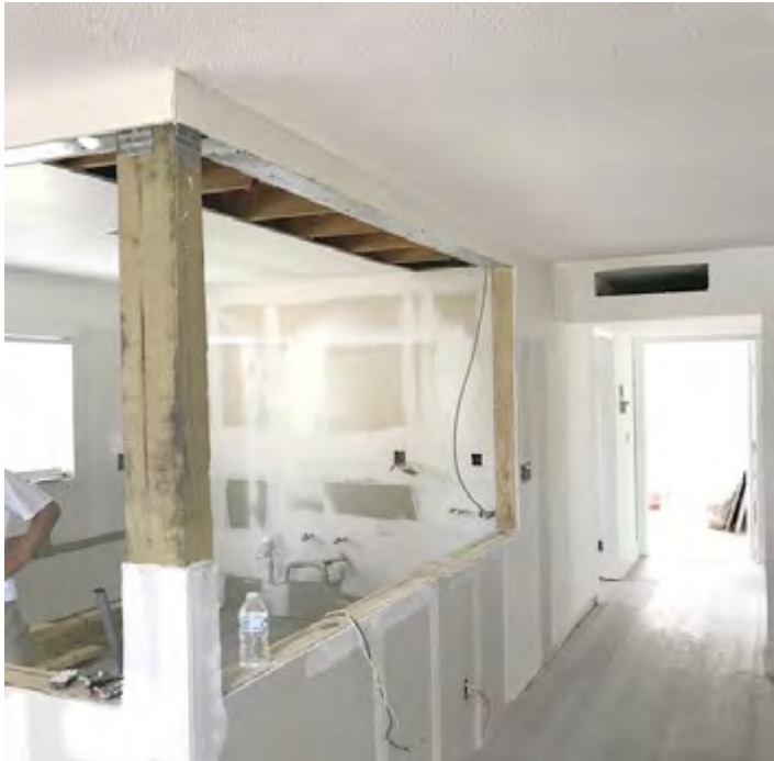
COVENTRY SECTION- THIS KITCHEN WALL IS (OR WAS) LOAD BEARING, MEANING THAT IT IS (WAS) HOLDING UP THE SECOND FLOOR. THE NEW WOOD POST AT LEFT IS INTENDED TO BEAR THE LOAD IN PLACE OF THE REMOVED WALL. WORK LIKE THIS IS TRICKY, AND NEEDS TO BE CAREFULLY DONE BY SKILLED TRADESMEN. A TEMPORARY SHORING BRACE WOULD HAVE KEPT THE CEILING FROM DROPPING DURING THE JOB.
