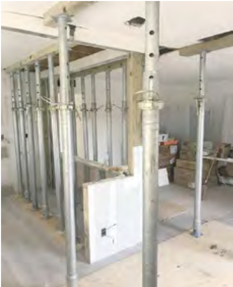
COVENTRY SECTION- AFTER THE CEILING DROPPED, THE UNIT OWNER INSTALLED FLOOR JACKS AND SHORED UP THE CEILING. TOO LITTLE, TOO LATE.
