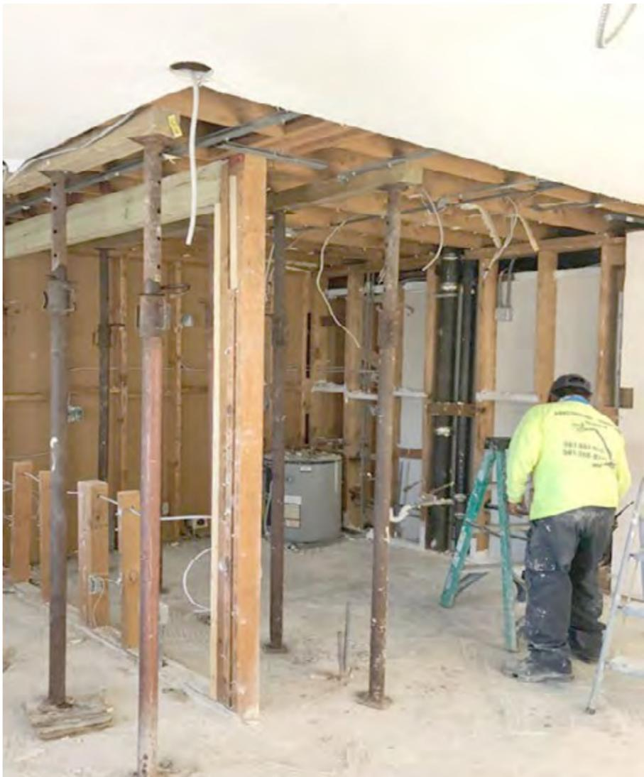
IN SOME BUILDINGS, INTERIOR WALLS ARE SUPPORTING MEMBERS, WHICH MEANS THAT THEY ARE HOLDING UP THE BUILDING. IN THIS CASE, REMOVAL OF FIRST FLOOR INTERIOR WALLS CAUSED THE SECOND FLOOR TO DROP. THE TEMPORARY SUPPORTS IN THIS PICTURE ARE HOLDING UP THE CEILING/FLOOR.
