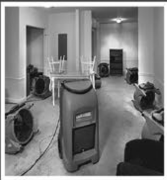
Structural Drying
