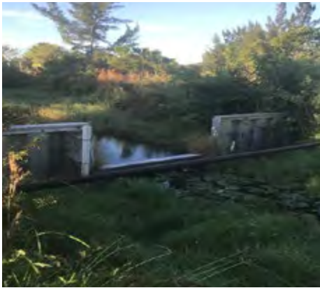
SOUTH LAGOON- THIS IS CV’S PRIMARY WEIR, A SMALL DAM WHICH HOLDS IN THE WATER OF ALL CV WATERWAYS. WHEN THE WATER LEVEL REACHES FOURTEEN FEET, WATER SPILLS OVER THE CENTER SECTION OF THE WEIR, AND MOVES TO CANALS OWNED BY LAKE WORTH DRAINAGE DISTRICT. THIS PICTURE WAS TAKEN ON 7/15; WATER IS JUST BARELY SPILLING OVER. I CALL THIS WIER “THE PLUG TO OUR BATHTUB”
