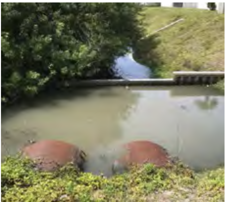
SOUTH CANAL, FAIRWAY STREET- THIS IS WHERE SOUTH CANAL CONNECTS WITH REFLECTION BAY. THESE TWO ROTTED OUT DRAIN PIPES WERE REPAIRED AND RE-LINED IN 2017.
