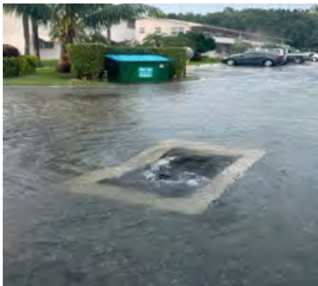
HASTINGS SECTION- THIS IS WHERE IT ALL STARTS. STORM WATER MOVES TO THESE CATCH BASINS, WHICH EMPTY TO UNDERGROUND PIPES THAT MOVE THE WATER TO OUR LAKES. FLORIDA RAINSTORMS ARE TORRENTIAL; DRAINAGE SYSTEMS ARE CRITICAL.
