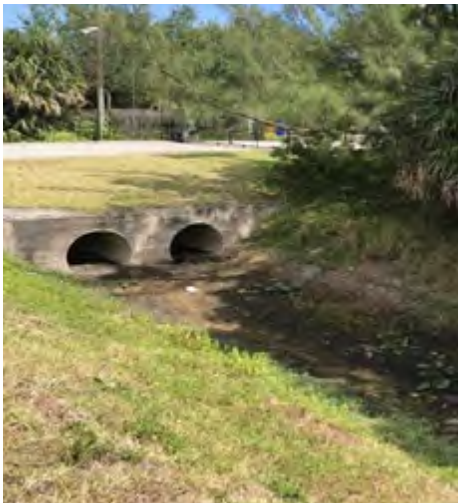
SOUTH CANAL- SECTIONS OF THIS WATERWAY HAVE BECOME FILLED IN OVER MANY YEARS, REDUCING ITS CAPACITY TO HOLD STORMWATER. THIS CANAL WILL BE DREDGED SOON.
