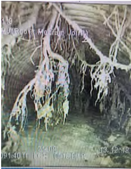
DURING THE TWO YEAR INSPECTION PROJECT, SOME SECTIONS WERE FOUND TO BE DAMAGED BY ROOTS. THESE SECTIONS WERE CLEARED AND REPAIRED.
