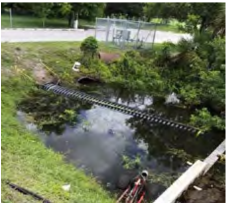
FAIRWAY STREET- THESE ROTTED OUT PIPES WERE RE-LINED WITH PVC INSERTS. THIS IS THE MOST COMMON WAY TO REPAIR DAMAGED UNDERGROUND DRAINAGE PIPES.
