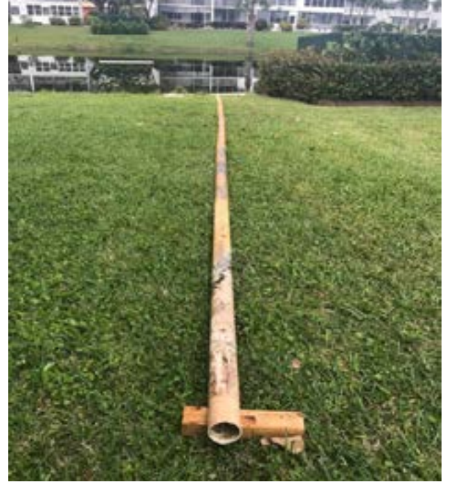
IRRIGATION WATER INTAKE PIPE- THESE NEED TO BE PERIODICALLY PULLED FROM LAKE AND CLEANED.
