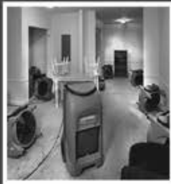
Structural Drying
